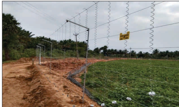
Hanging Type Solar fencing system installed in the farmer's field
